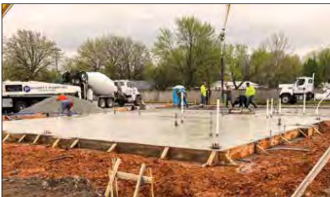
Workers level the slab as construction begins on the new Myaamia National Archives
