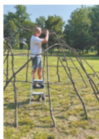
Lashing saplings together in building a wiikiaami. Photo by Joshua Sutterfield.
