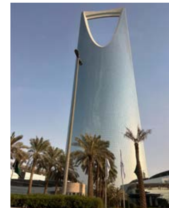
One of many skyscrapers in Riyadh, that offers an amazing view of the city from the "skybridge." Photo by Logan York.
