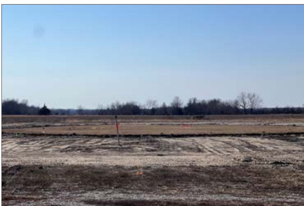
Removal of sidewalk progress. Photo by Madalyn Richardson, MTO.
